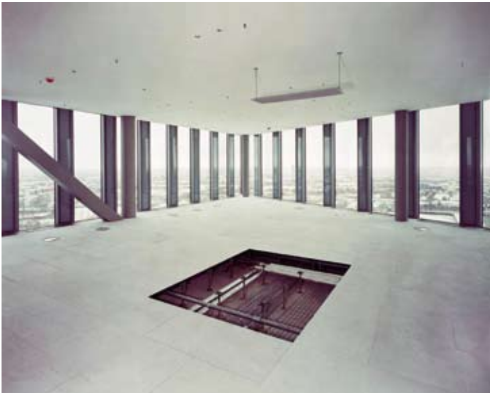
MERO-TSK Hollow Floor (600x1200 mm) at Munich Tower
